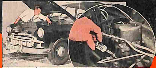
Car owner making one-minute adjustment of carburetor idling screw for more gas mileage. He will also clean spark plugs and set points to prescribed clearance. Then by following simple gas-saving driving rules and other common sense ways to save on gas, he'll save up to $50.00 a year on gasoline alone!
