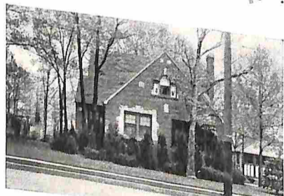
Home of Mr. and Mrs. J. D. Wiert, Rockville Centre, Long Island
