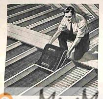
Fits Like a Glo attic. Simply fasten one end of KIMSUL ... stretch it taut and fasten to opposite eave. Repeat for each open section. That's all! If your attic is floored, apply Kimsur-between the rafters of your sloping roof.
