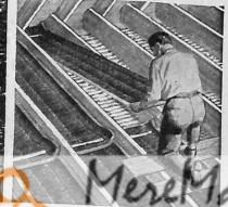
44† Layers in One Blanket - With 44 separate layers of insulation backed with heavy water-proof paper and stitched together, KIMSUL is scientifically superior to loose, bulk insulation in these ways: (1) Provides uniform protection over every inch of insulated area. (2) Retains original thickness - no sagging, sifting,
