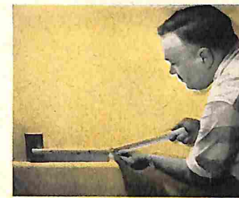
New electric outlets made easy! These strips screw to the wall to put 'em where you want 'em
